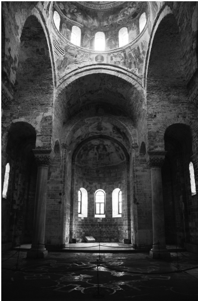
FIGURE 21.1. Hagia Sophia church (between 1238 and 1263), Trebizond, interior looking east. Domed nave of the cross-in-square type with sanctuary apse. Photo: Nebojša Stanković.
